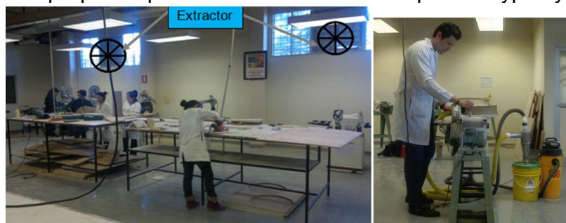
Figure 5. General and localized, ventilation to improve air and provide comfort in laboratory
